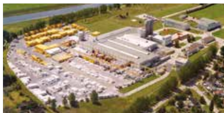
Calbe Factory, Germany
