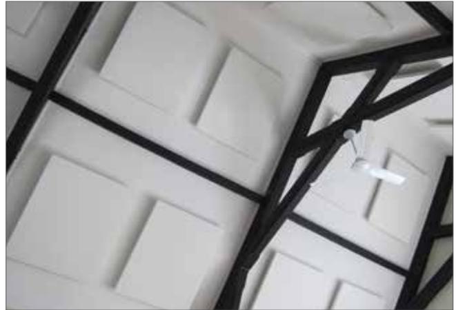
with built in support frames to allow for bracket fixing to provide an air void behind the absorber for enhanced acoustic performance.
