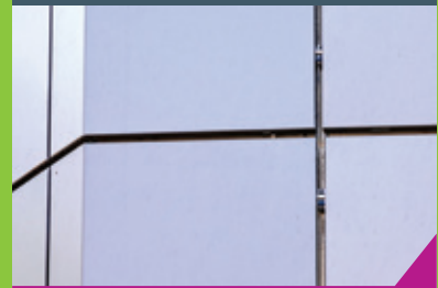
Typical Metal Façade
