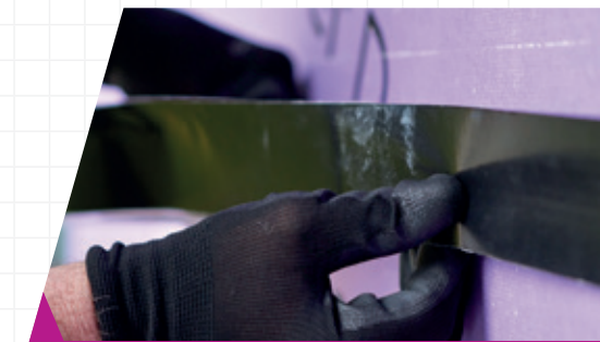
Weather Defence Joint Tape being applied
